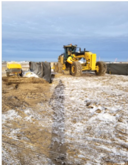
Oct 15/18 Description & Location KP- 884+072 Photo taken west. Grater waiting for workers to blow any debris that is on machine before it can cross road at SF 51
